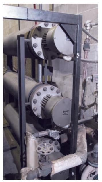
Cleaning the Vitafoam system "on the fly" involved draining used heat transfer fluid from the heat exchanger and replacing it with the Paratherm LC™ system cleaner. Production continued while the system was cleaned. After 4 weeks the system was drained and recharged with Paratherm NF® heat transfer fluid.
